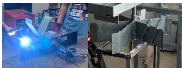
Fig. 2b Fabrication of Turbine blades with welded rebar as fins
